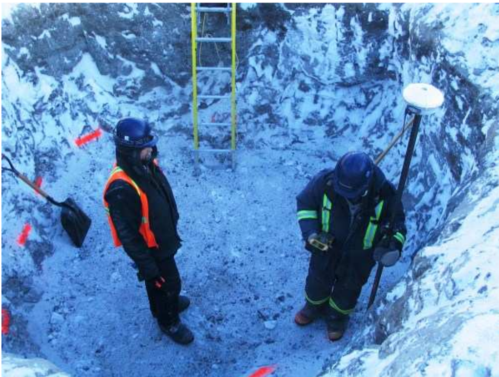
Photo 4: Sump 2 with snow removed. Surveyor marking 5/8 clear levels.
