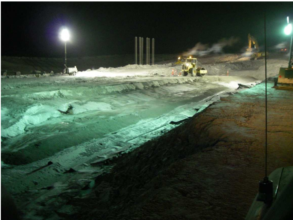
Photo 12: View of the lift of material placed along the upstream edge of the core. The compactor is parked at the edge of material placed in the north square. Photo taken from Sta. 1+20 looking north.
