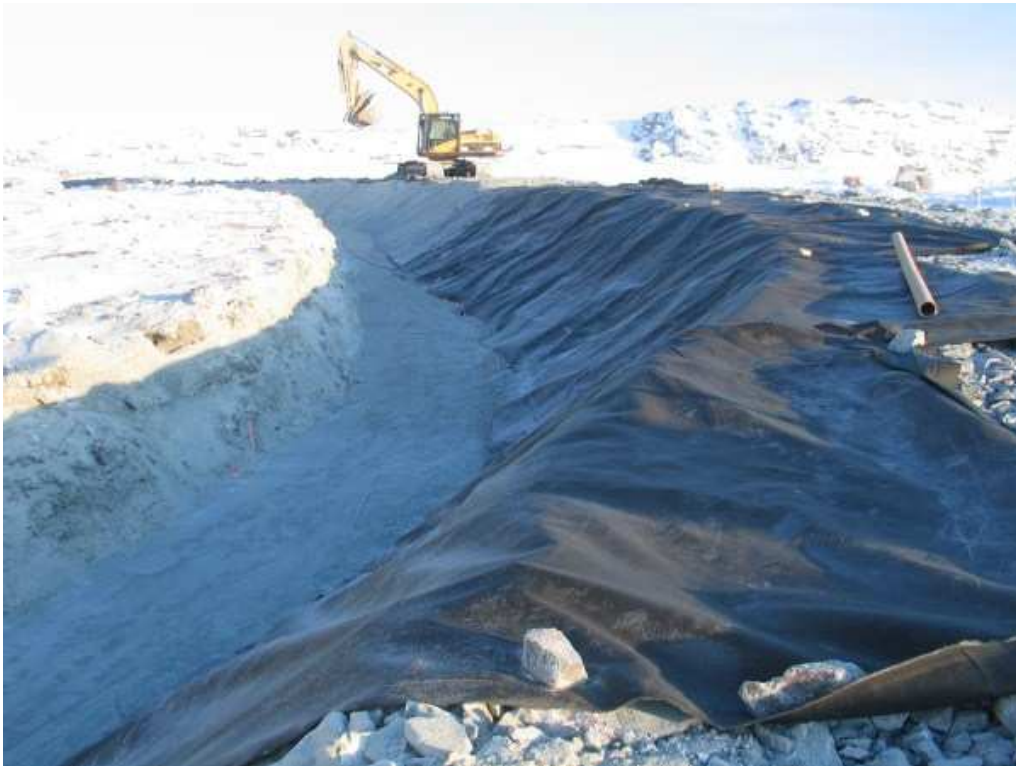
Photo 11: Underliner placed to Sta 0+340.
