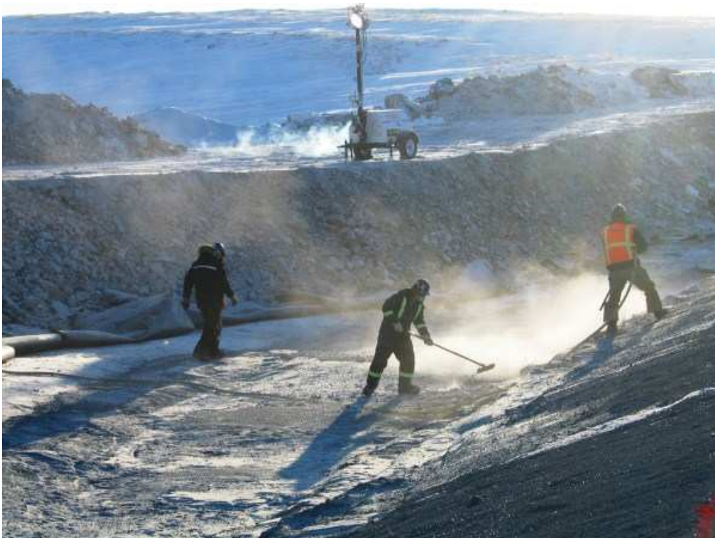
Photo 8: Cleaning in the extended fillet area with air compressor.
